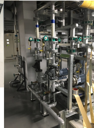
Water cooling facility has been already expanded in our data center building.
