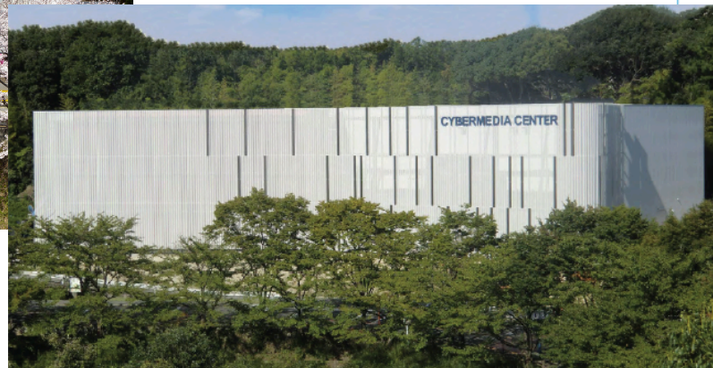
IT Core Annex: new datacenter building
